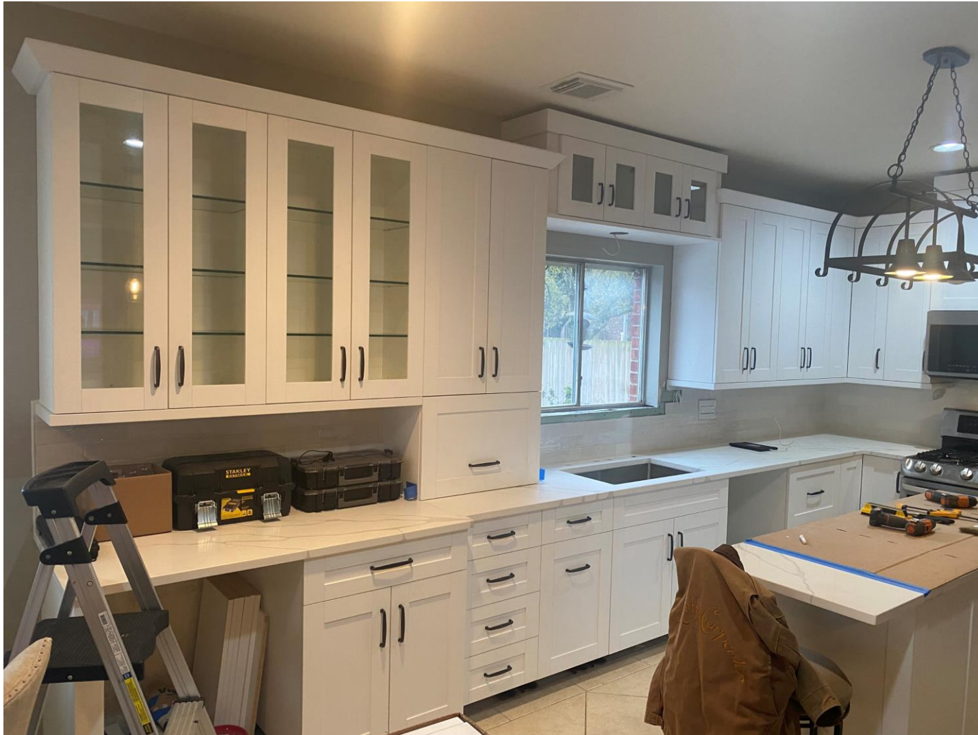
SHIFT DS5 WINTER FOREST FACTORY INSTALLED CLEAR GLASS (SHELVES BY OTHERS) -WALL APPLIANCE GARAGE WITH SWING UP DOOR
